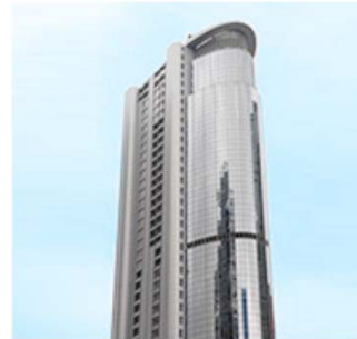
EXCEL ELECTRONICS (HONG KONG) LTD.
